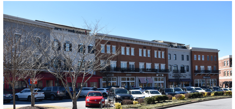
Image 13. Building facades at Suwanee Town Center
