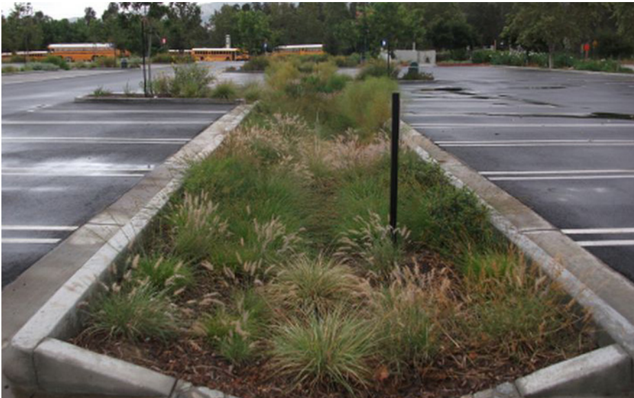
Image 18. Bioswale located at the Los Angeles Zoo Parking Lot
